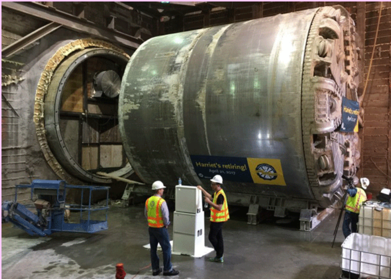
Harriet the Tunnel Boring Machine ready to retire-front view!
